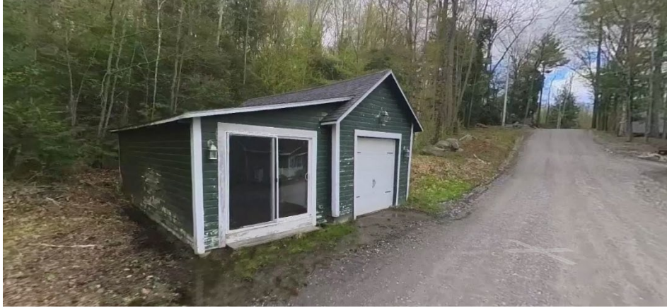
Google Maps Image 1 (dated 11/26/2025): Google image on Burma Road looking south. The existing structure is between 14 feet and 17 feet from the ROW; the proposed structure would be located 20 feet from the ROW (Google, May 2024).
