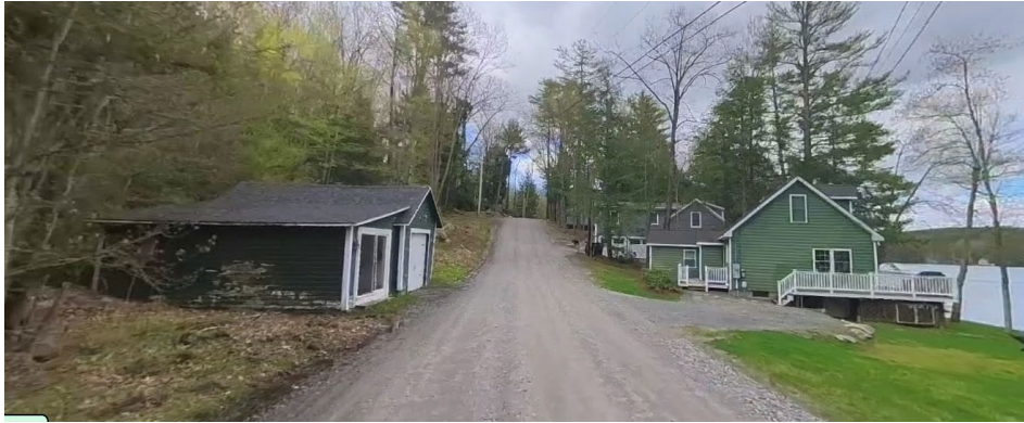
Google Maps Image 2 (dated 11/26/2025): Google image on Burma Road looking south. The existing structure is between 14 feet and 17 feet from the ROW; the proposed structure would be located 20 feet from the ROW (Google, May 2024).
