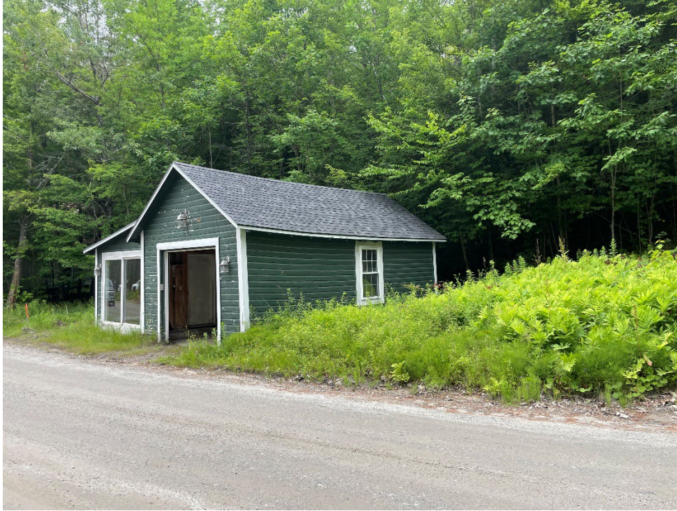
Photograph No. 1 (dated 07/11/2025): View looking northeast on Burma Road at the existing garage structure. The structure is not parallel to Burma Road. The front of the structure is between 14 feet and 17 feet off the right-of-way (ROW). The proposed structure would be located 20 feet off the ROW. The abandoned wastewater system is to the right (south).
