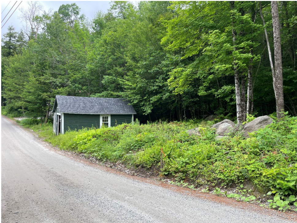
Photograph No. 2 (dated 07/11/2025): View looking north on Burma Road at the existing garage structure. The property's south boundary marker can be seen in the ROW to the left of the boulders.
